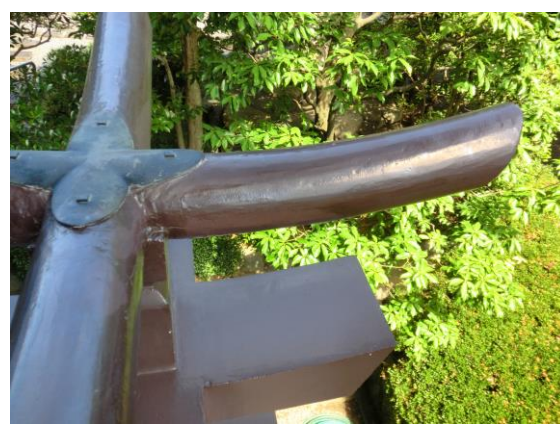
修理跡を塗装
