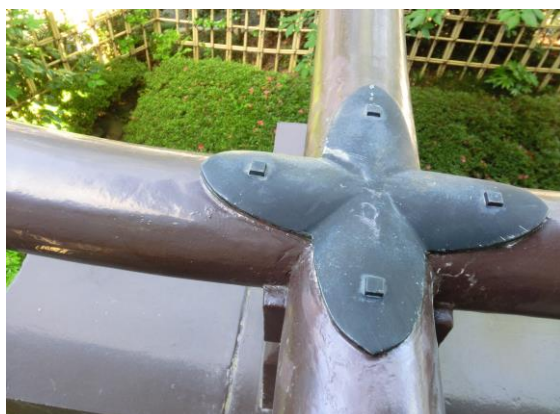
修理跡を塗装
